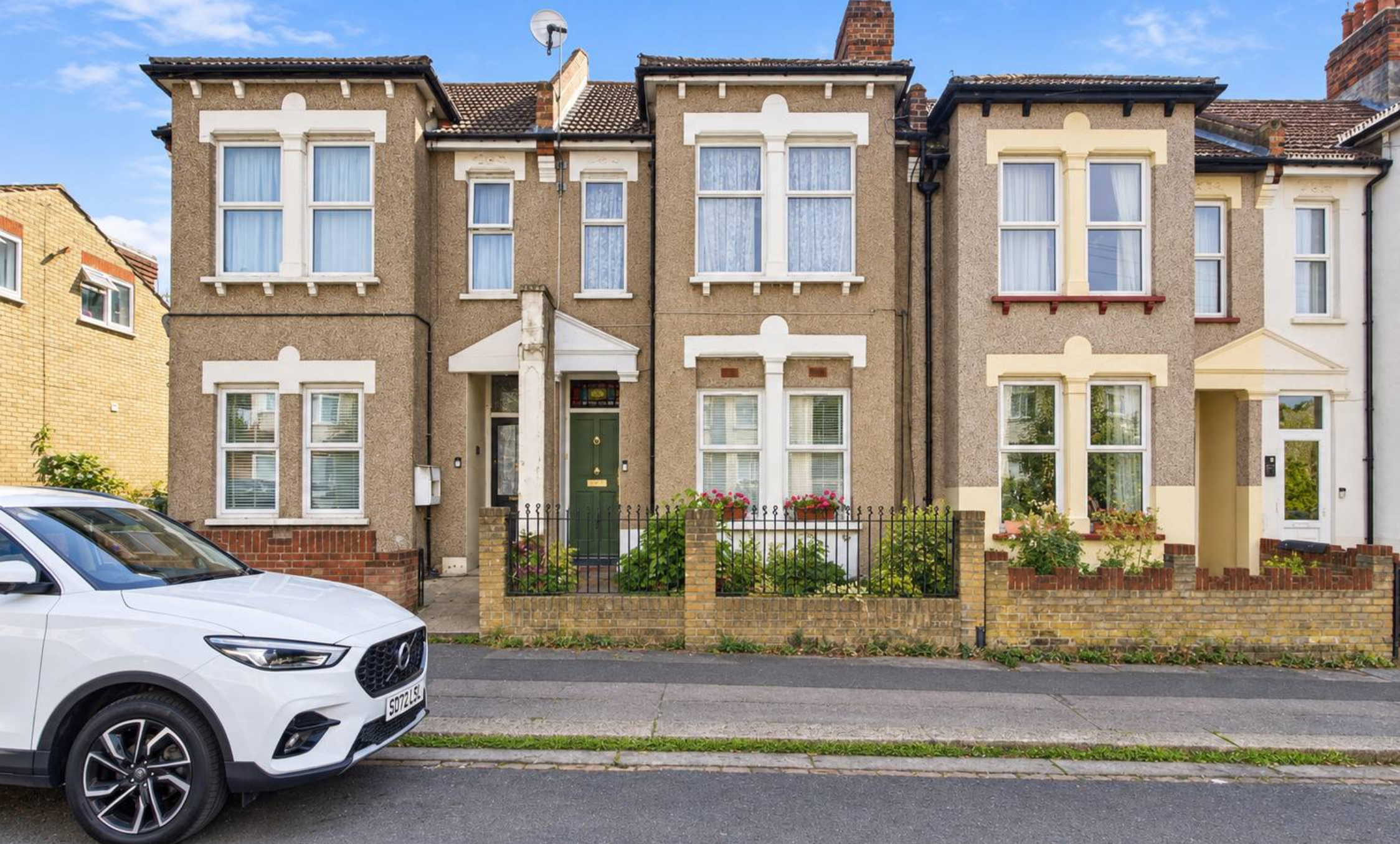
118 Burlington Road, Thornton Heath £350,000
