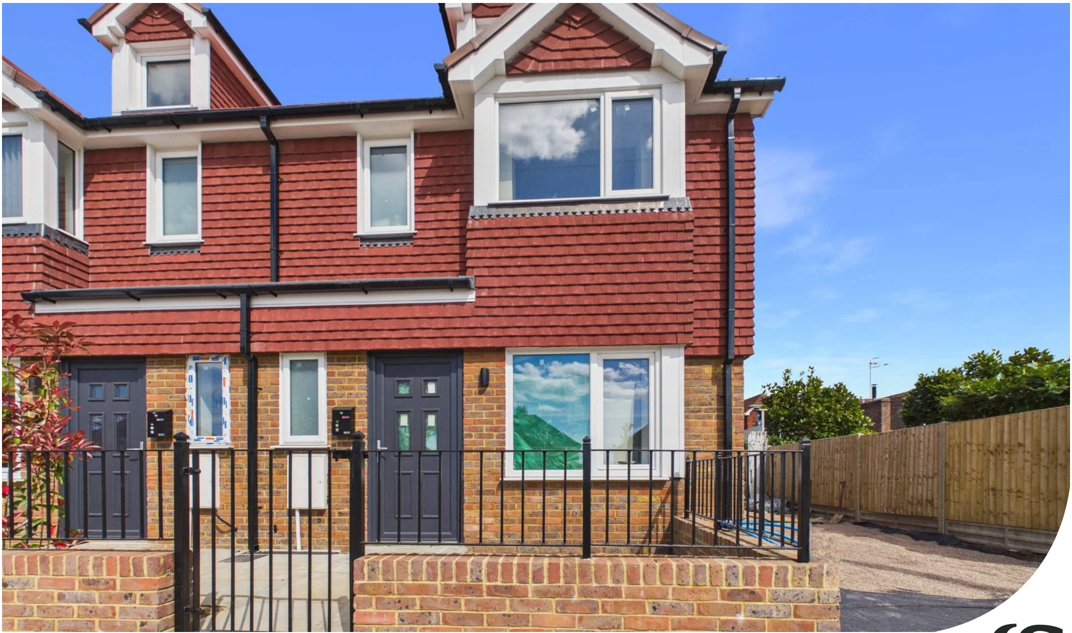
Upper Shoreham Road, Shoreham by Sea £475,000
