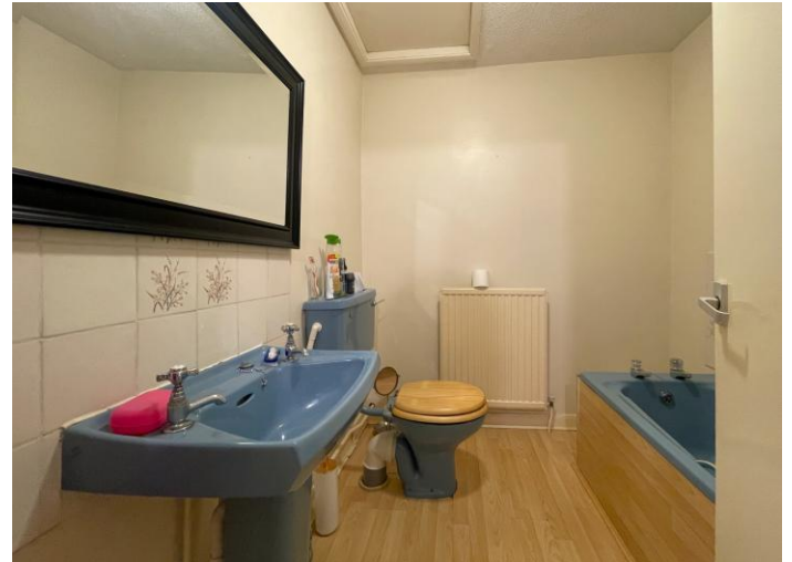
Bathroom - Basement Flat (1)
