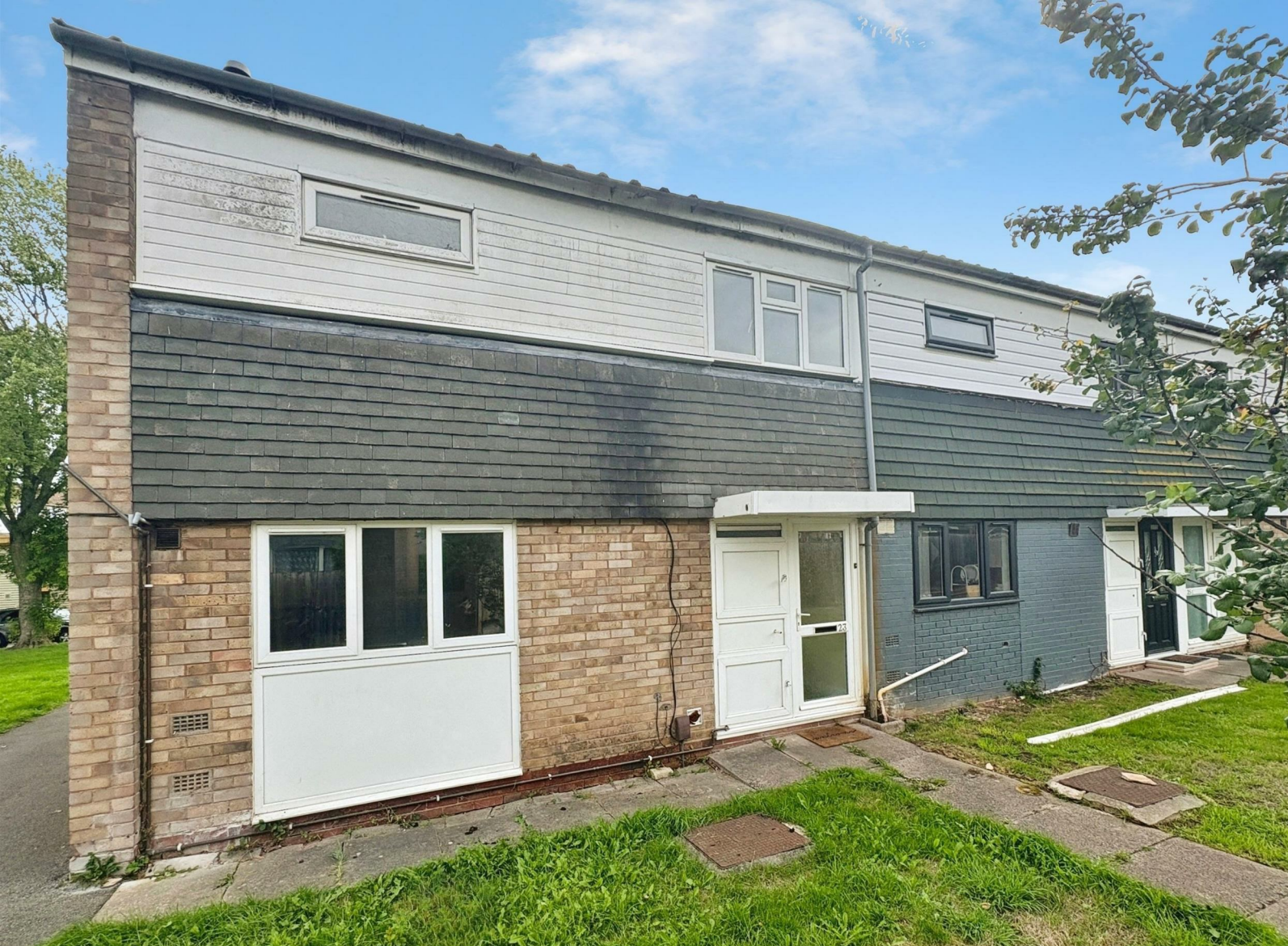
Eckington Close, Redditch
