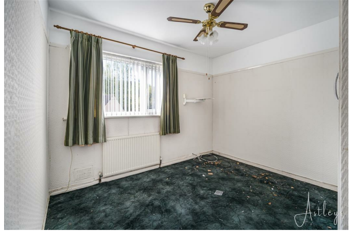
Storage cupboard, radiator and window to the front
