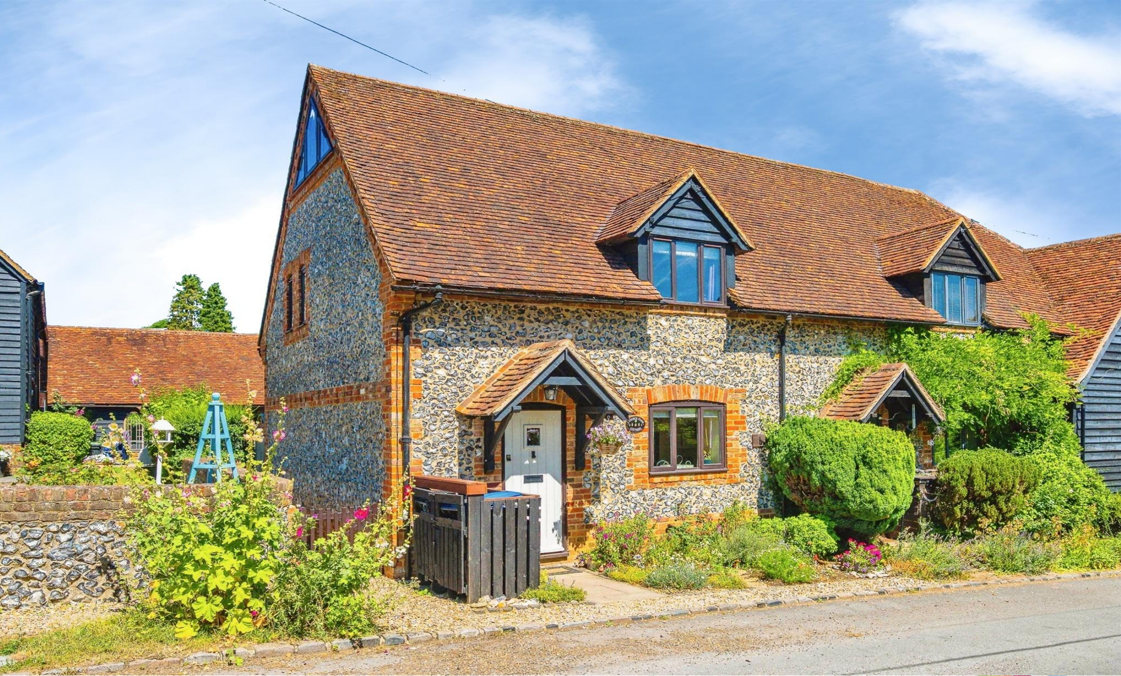
Church Farm Cottages Pipers Hill, Great Gaddesden HEMEL HEMPSTEAD HP1 3BY
