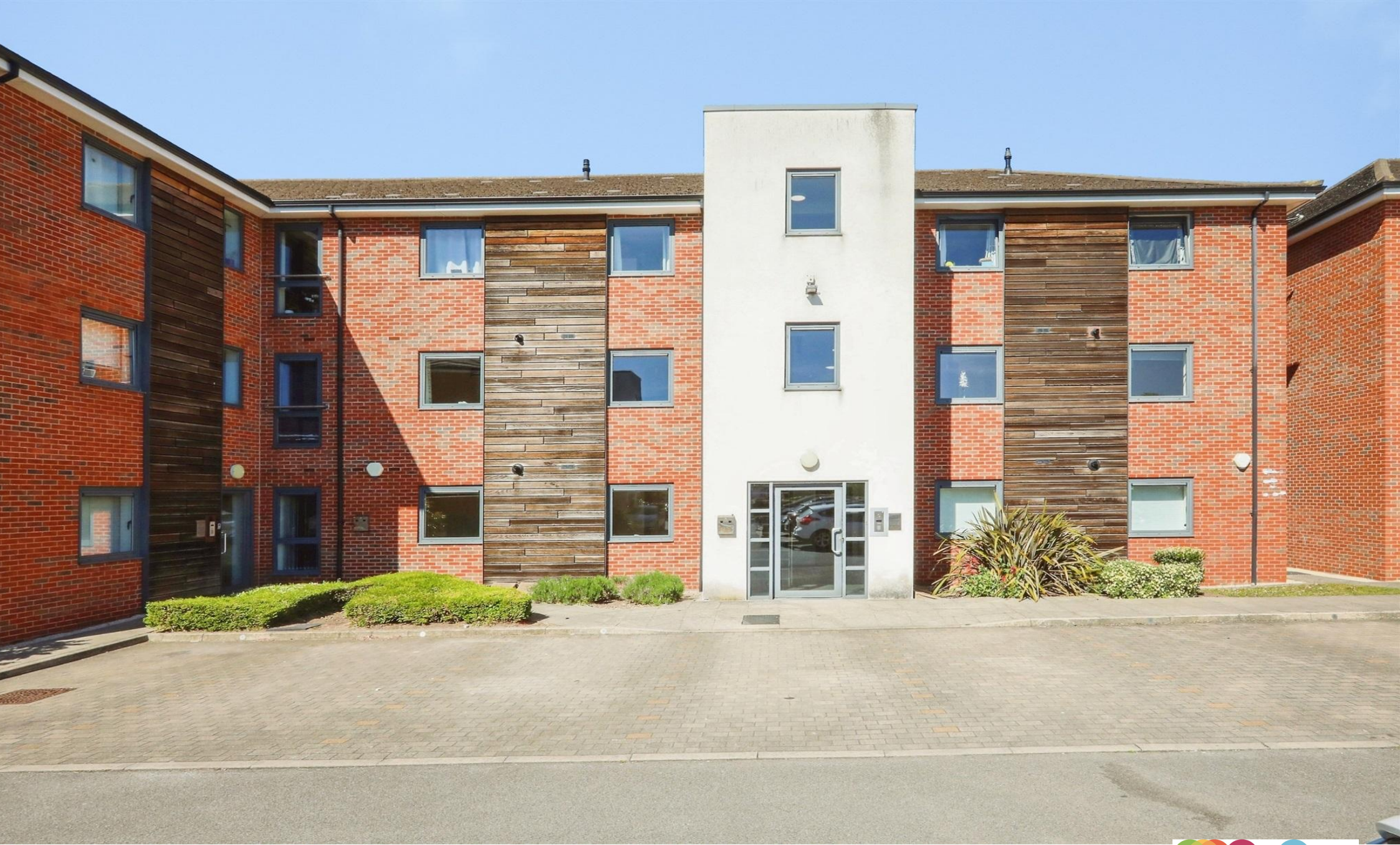
Rectory Court Mere Lane, Armthorpe Doncaster
