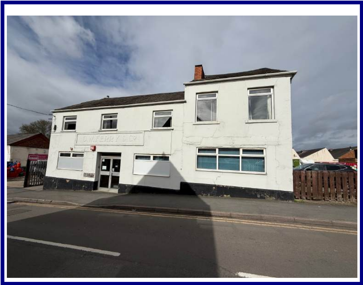
Office building access from Stockwell Head
