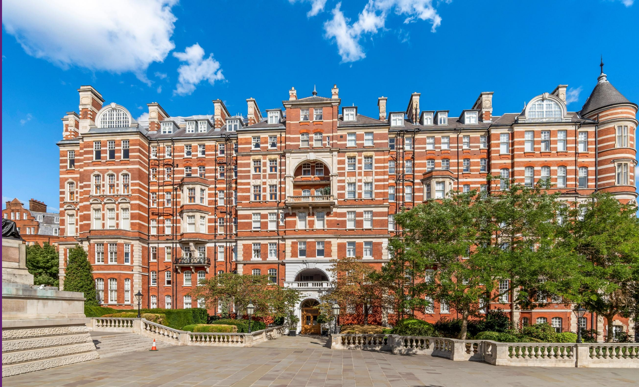
Albert Court West Block Prince Consort Road, SW7
