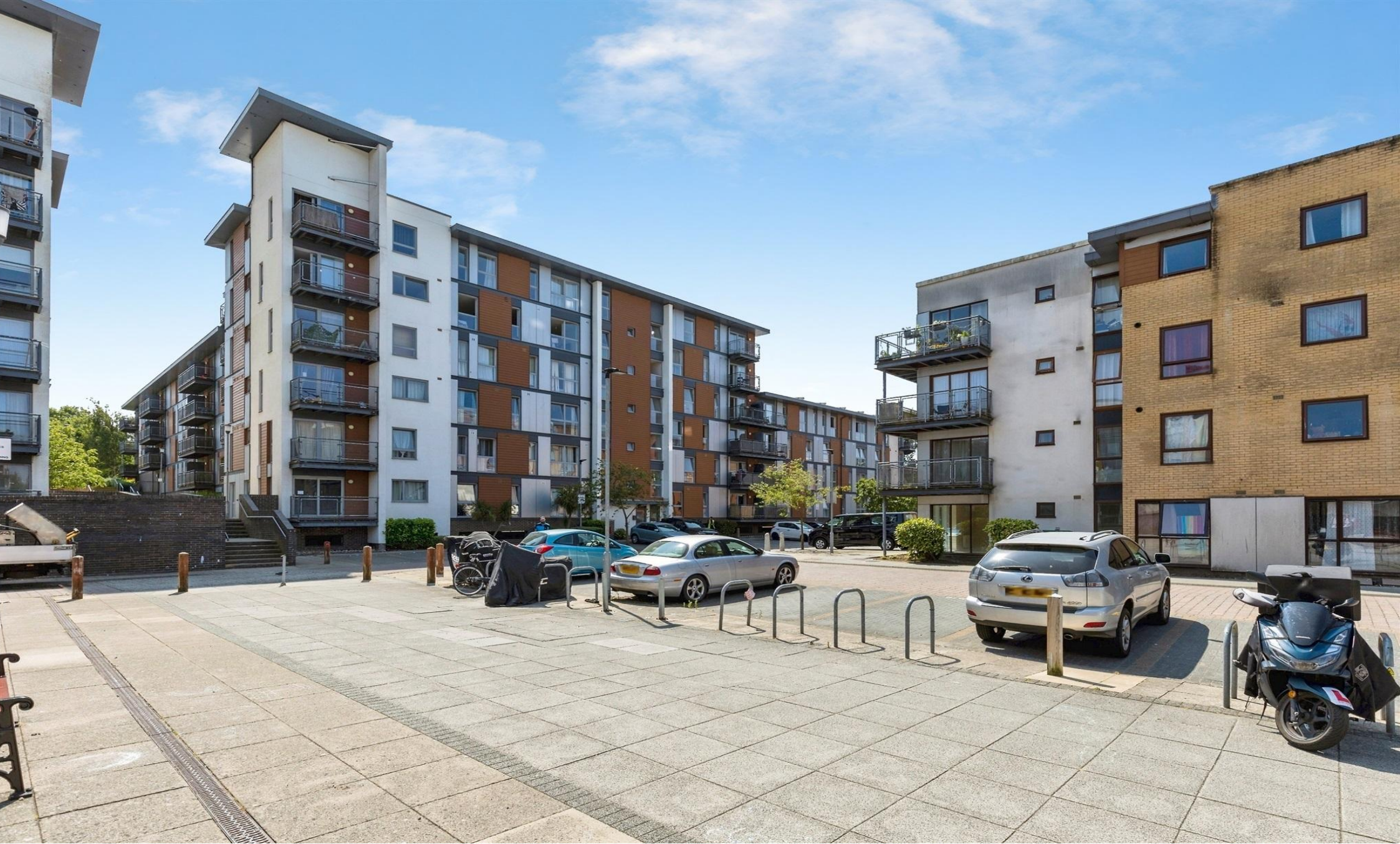
Page Court Commonwealth Drive, Crawley RH10 1AR
