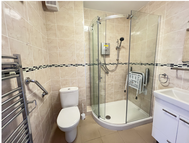
REFITTED SHOWER ROOM with low level w.c., vanity wash basin, tiled and glazed shower cubicle with thermostatic control, extractor fan, tiled walls, electric towel rail radiator, tiled floor and Dimplex heater.
