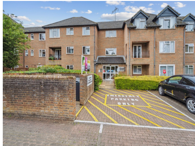
To the front there is ample visitor and resident's car parking areas, bin storage and laundry courtyard.
