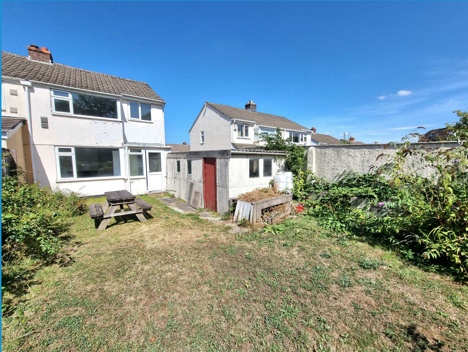
St. Johns Road Launceston | Cornwall
