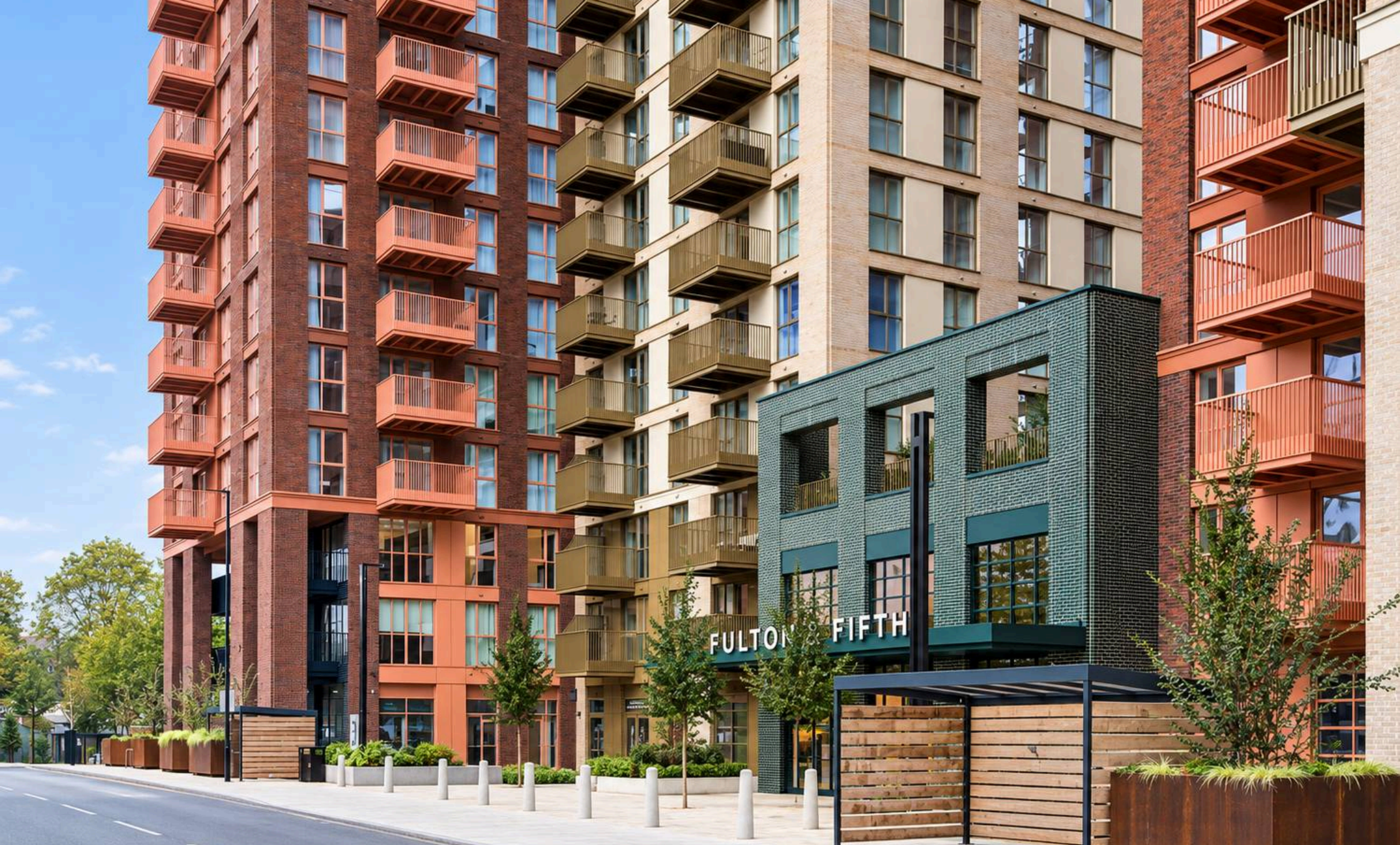
Brookline Building, Fulton Road, Wembley
