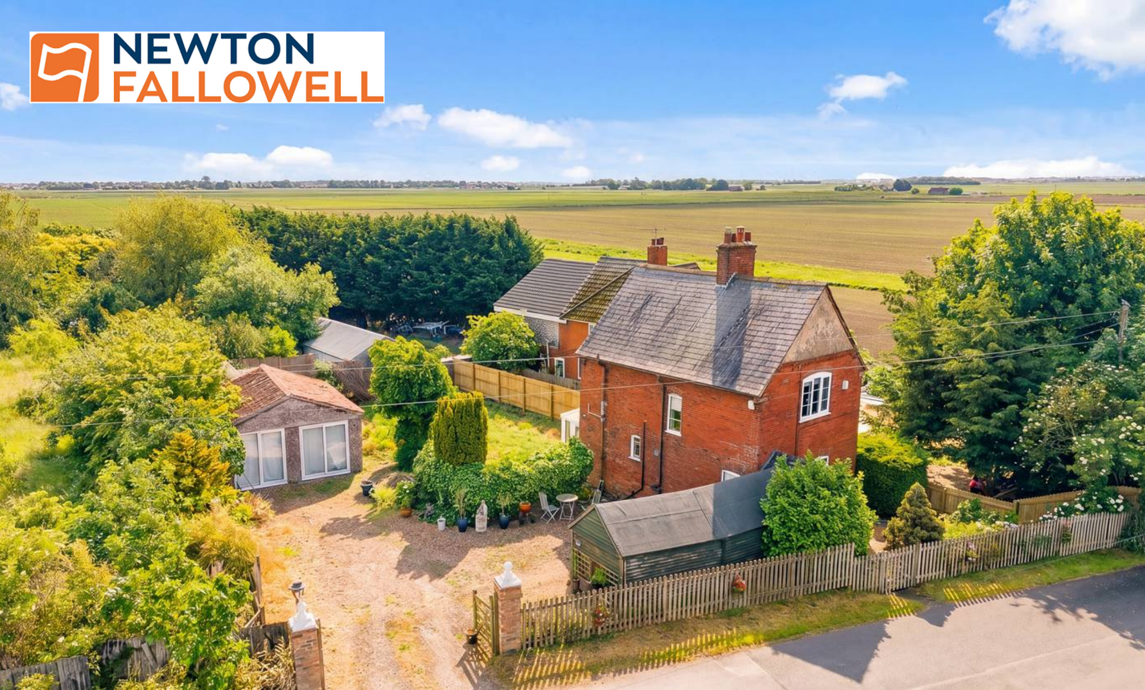
Station Crossing Cottage, Station Road, Stickney – PE22 8HW £250,000
