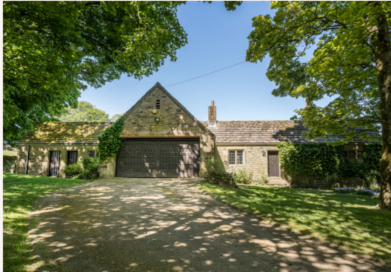
GARAGE & BENTS COTTAGE
