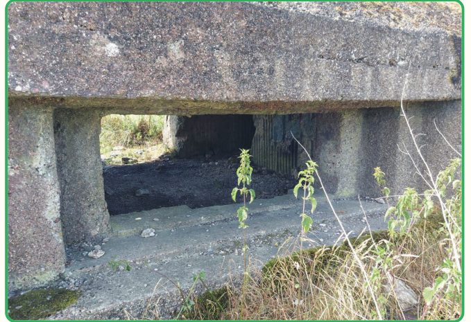
INTERIOR THROUGH THE OPENING
