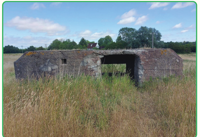
ACCESS OPENING, LOOKING TOWARD THE VILLAGE
