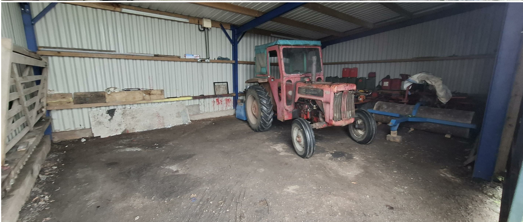
Agricultural Storage Building 30'6" x 19'11" (9.29m x 6.06m) Steel frame and sheeted build
