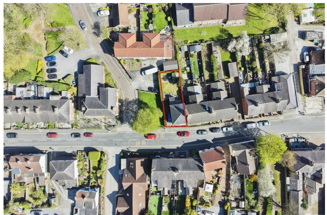
Aerial view of the property
