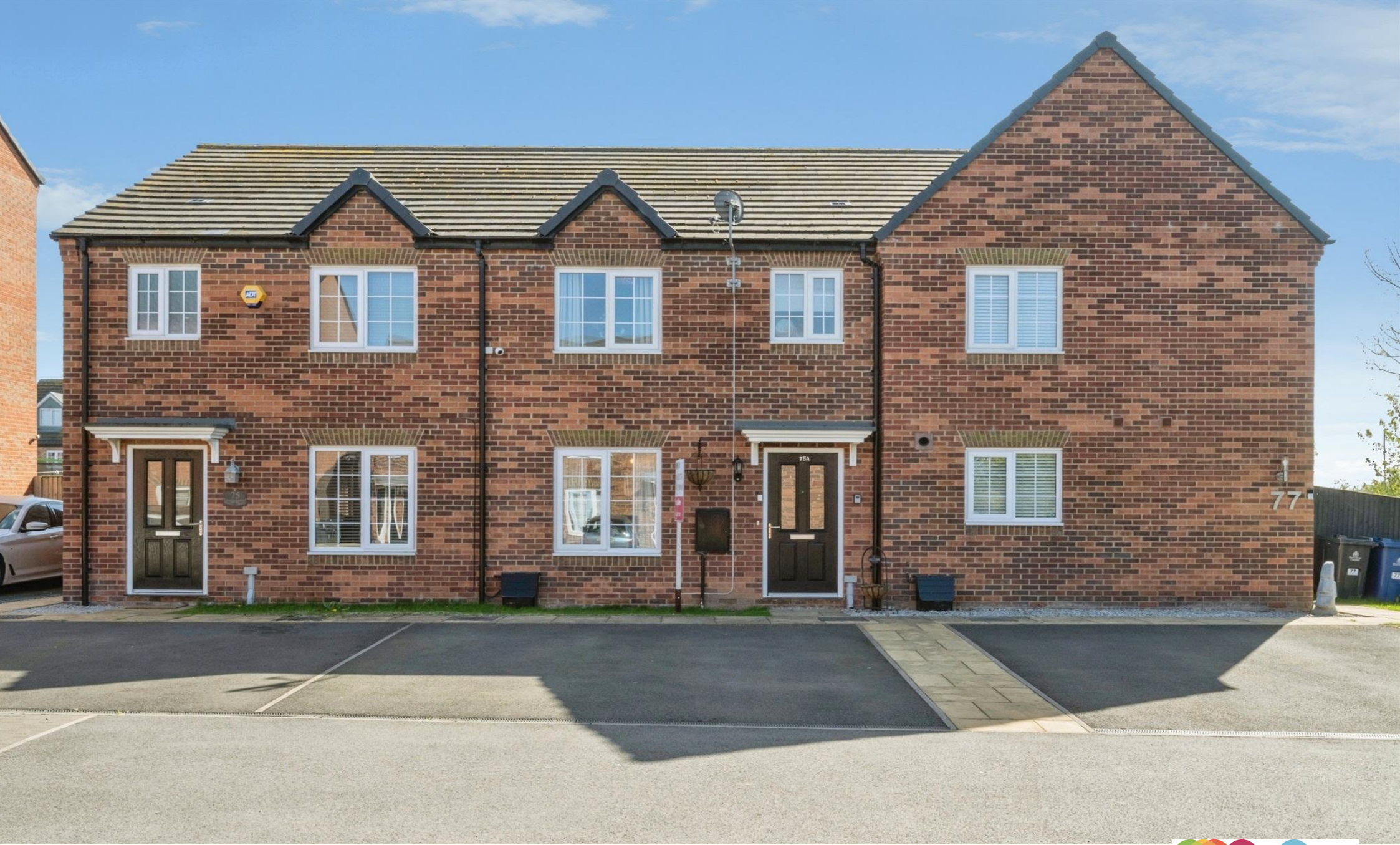
Heatherfields Crescent, New Rossington Doncaster
