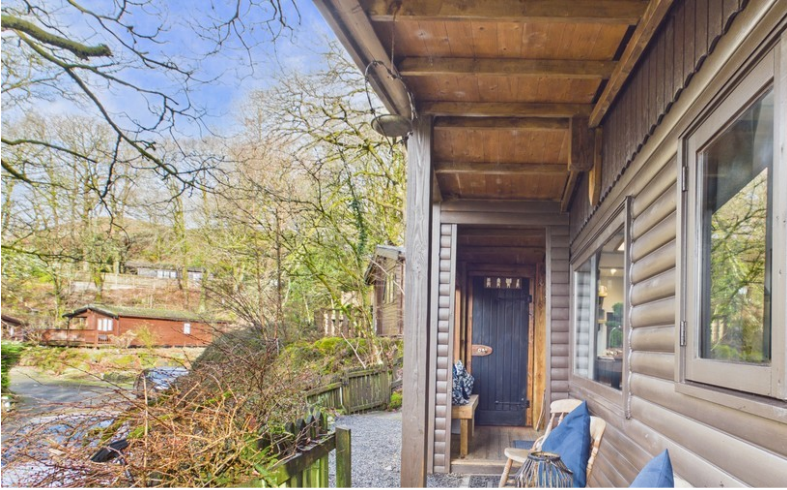
Covered Seating Area
