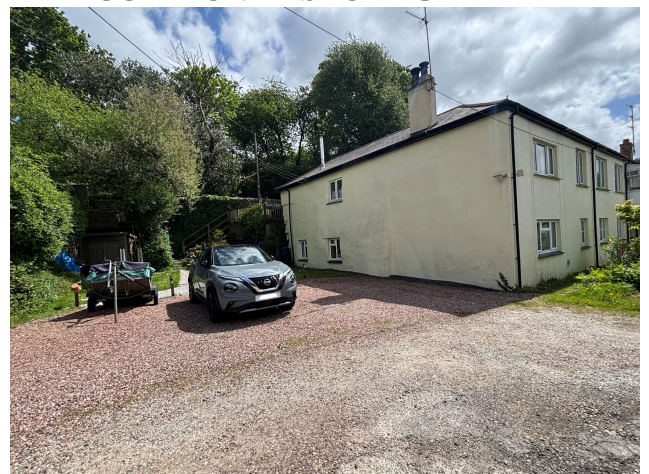
PARKING AREA TO THE REAR
