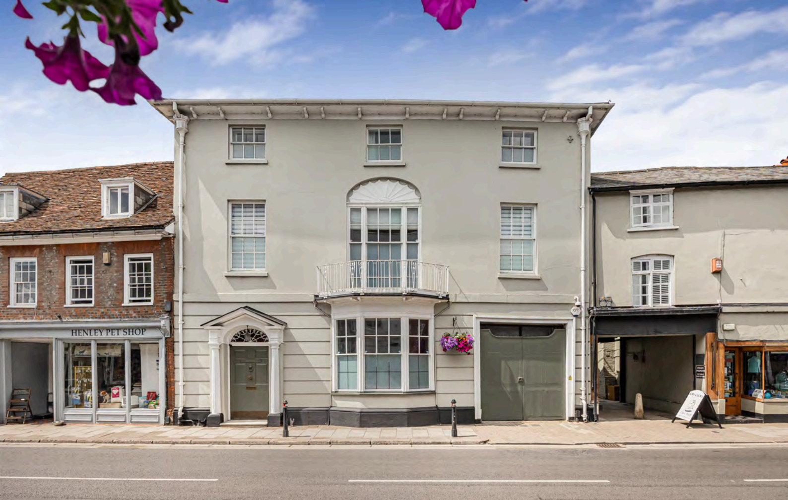
ADAM HOUSE, BELL STREET, HENLEY-ON-THAMES
