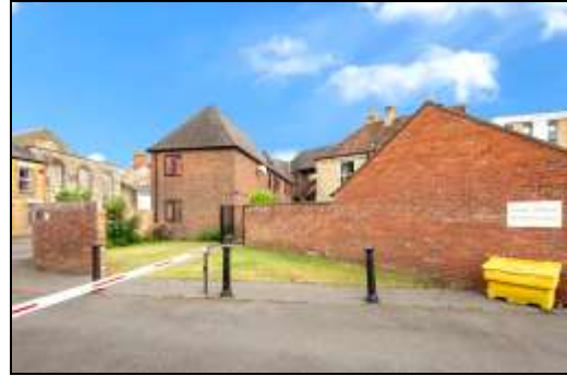
Barrier Controlled Car Parking Area
