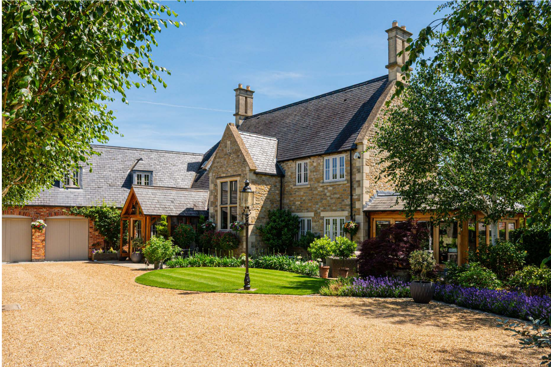
Butlers Manor, Pytchley Road, Orlingbury
