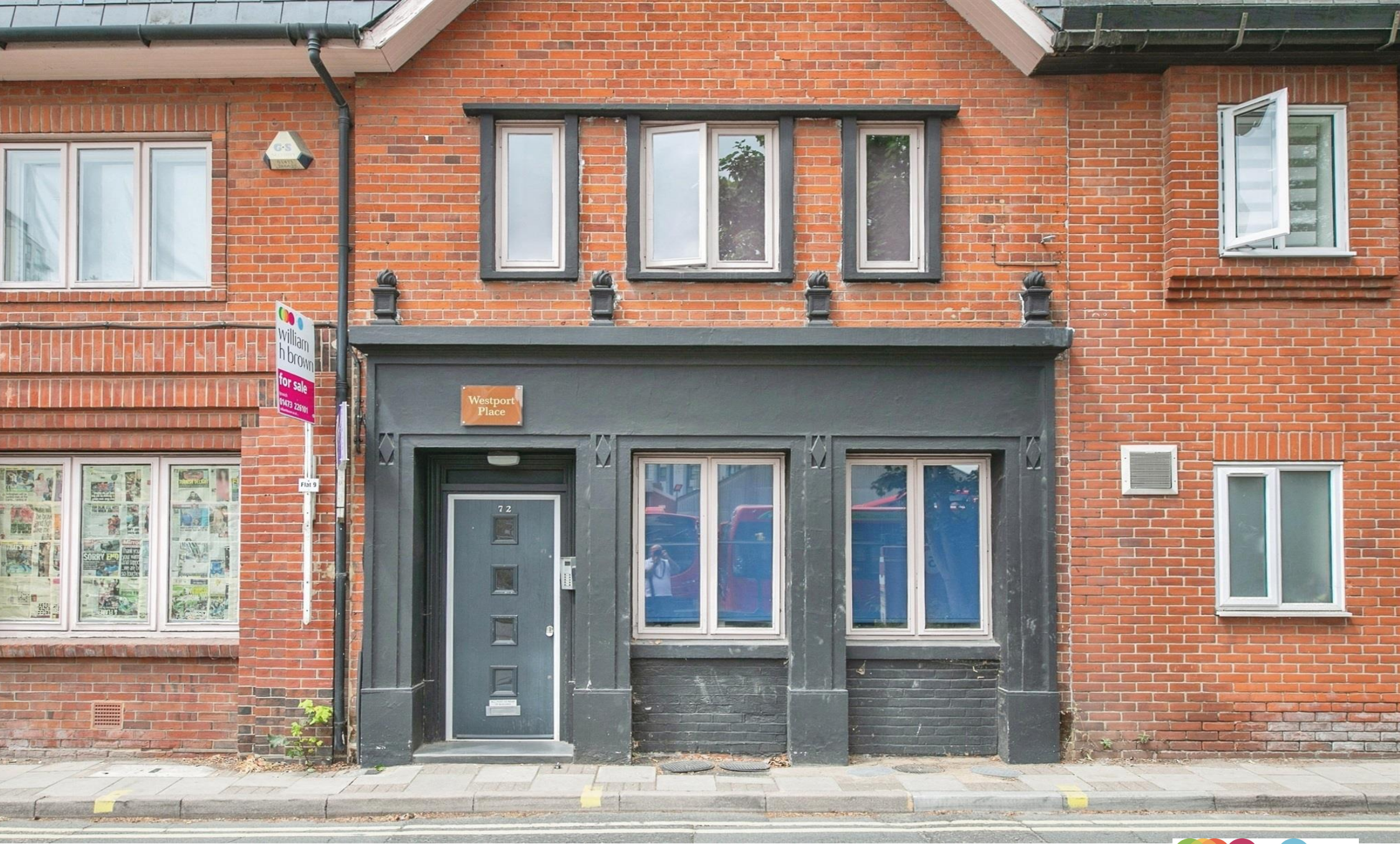
Westport Place, Foundation Street, Ipswich, IP4 1BN
