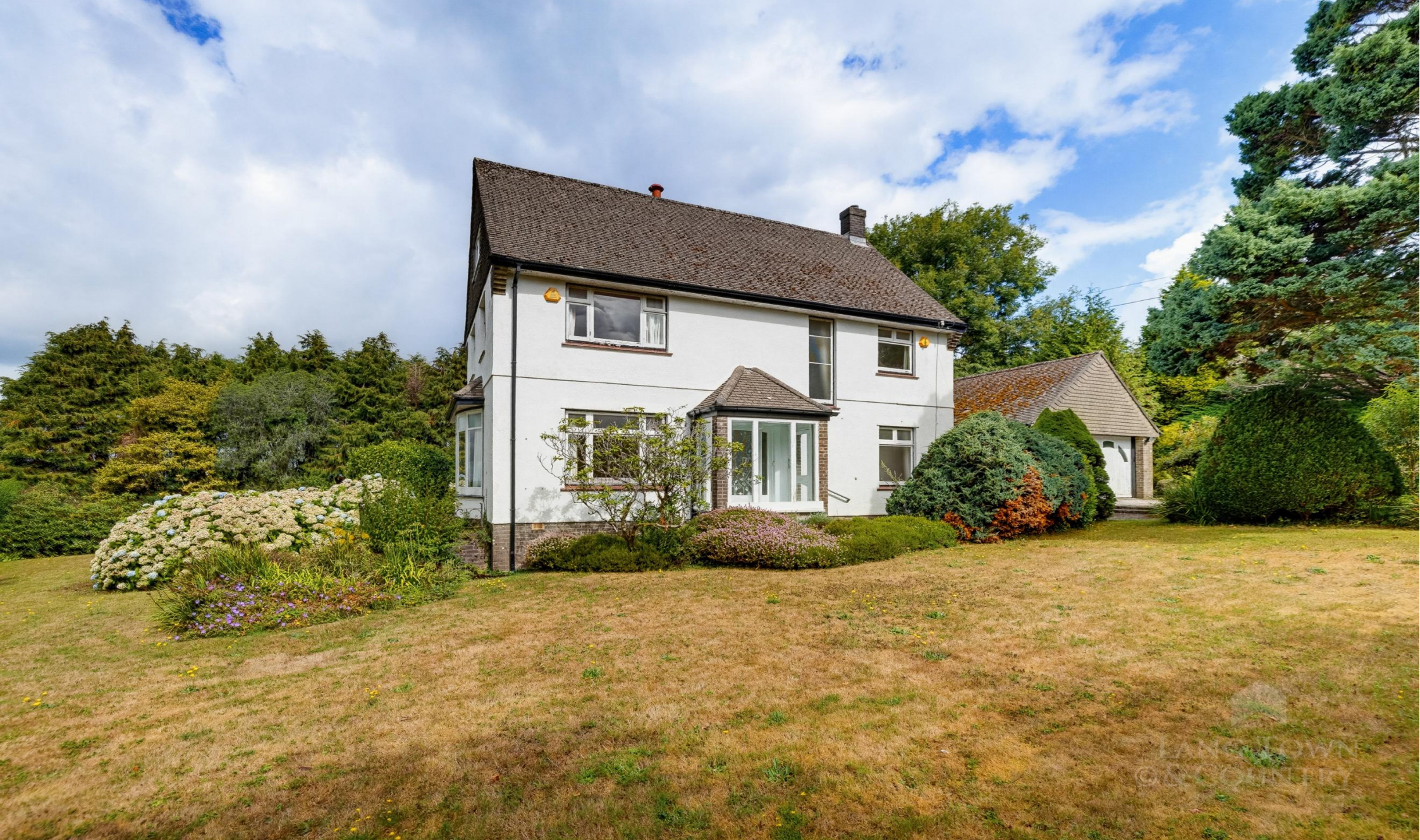
The White House, Green Lane, Yelverton, Devon, PL20 6BW
