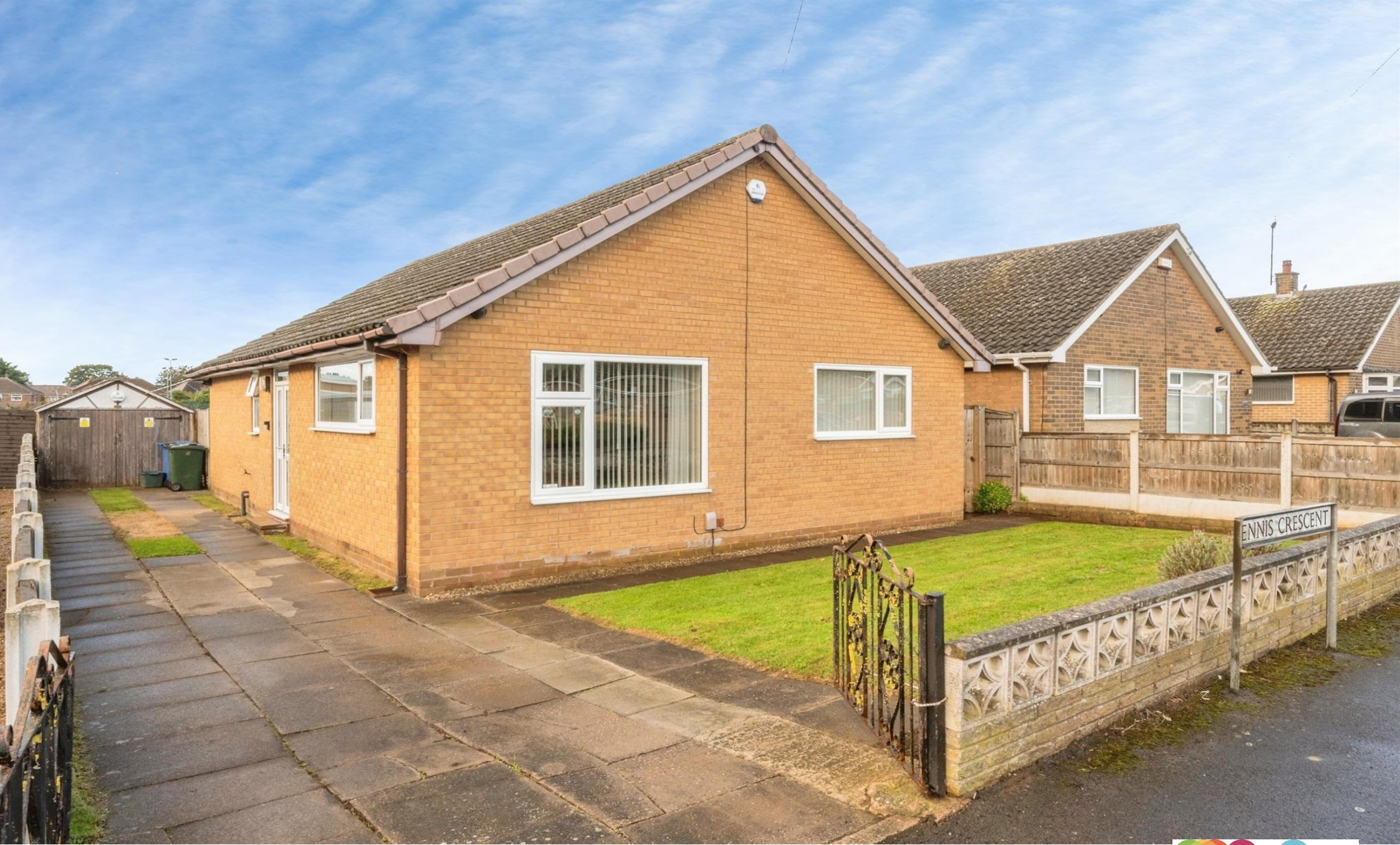
Ennis Crescent, Intake Doncaster
