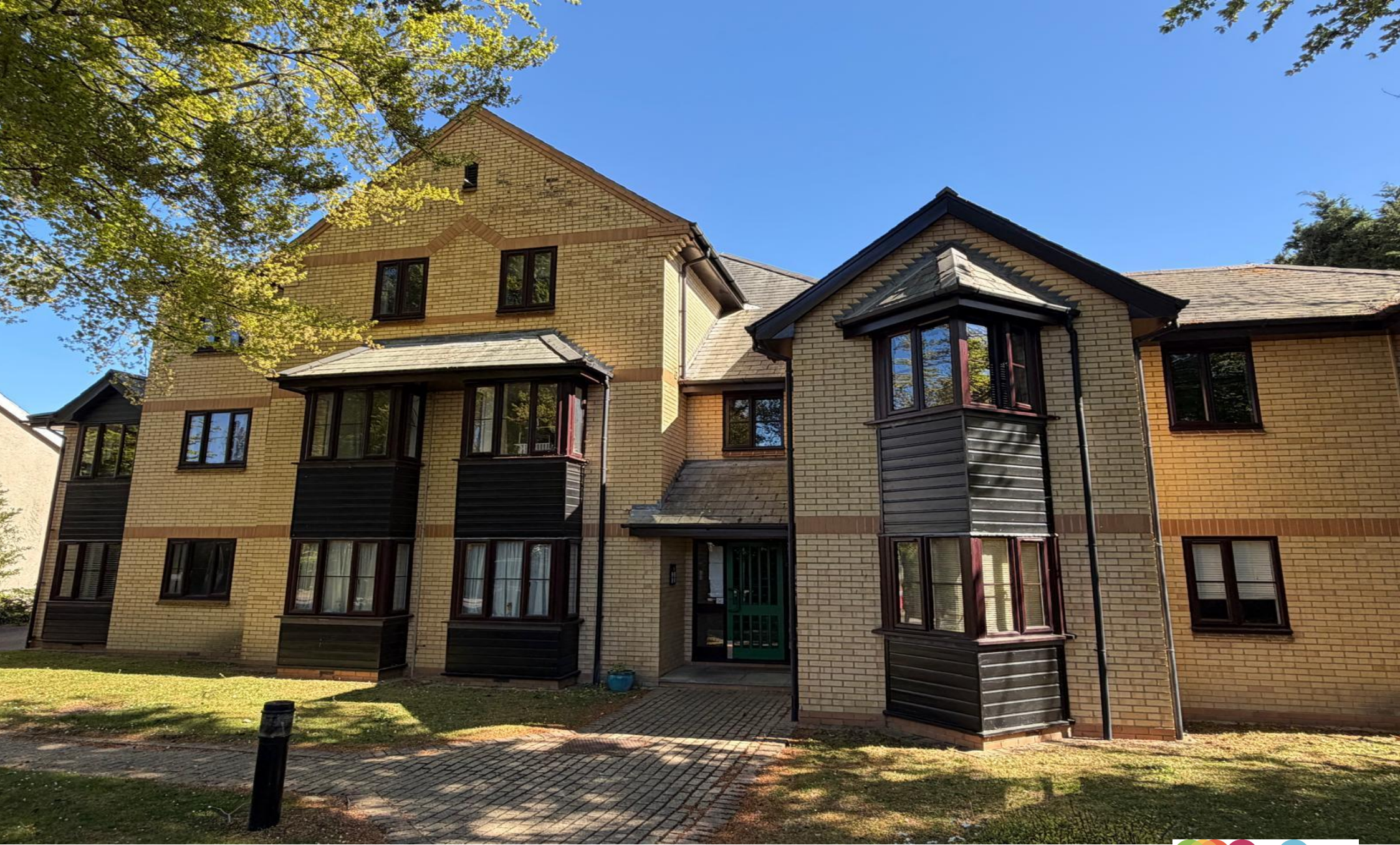
The Beeches, New Road, Melbourn, SG8 6BX
