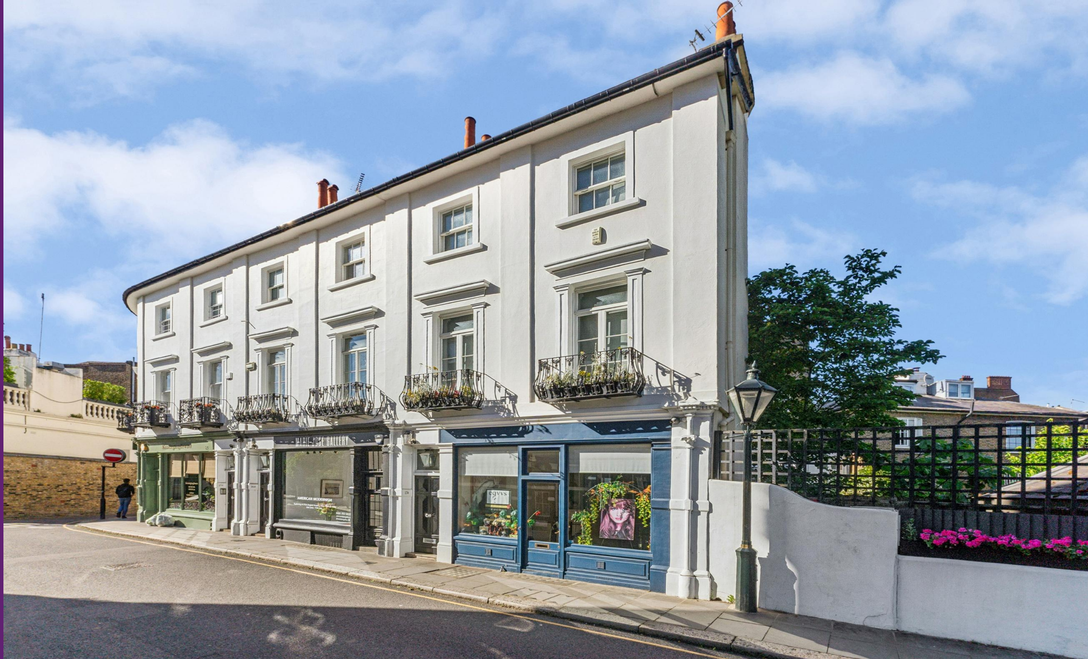
Victoria Grove Kensington, W8
