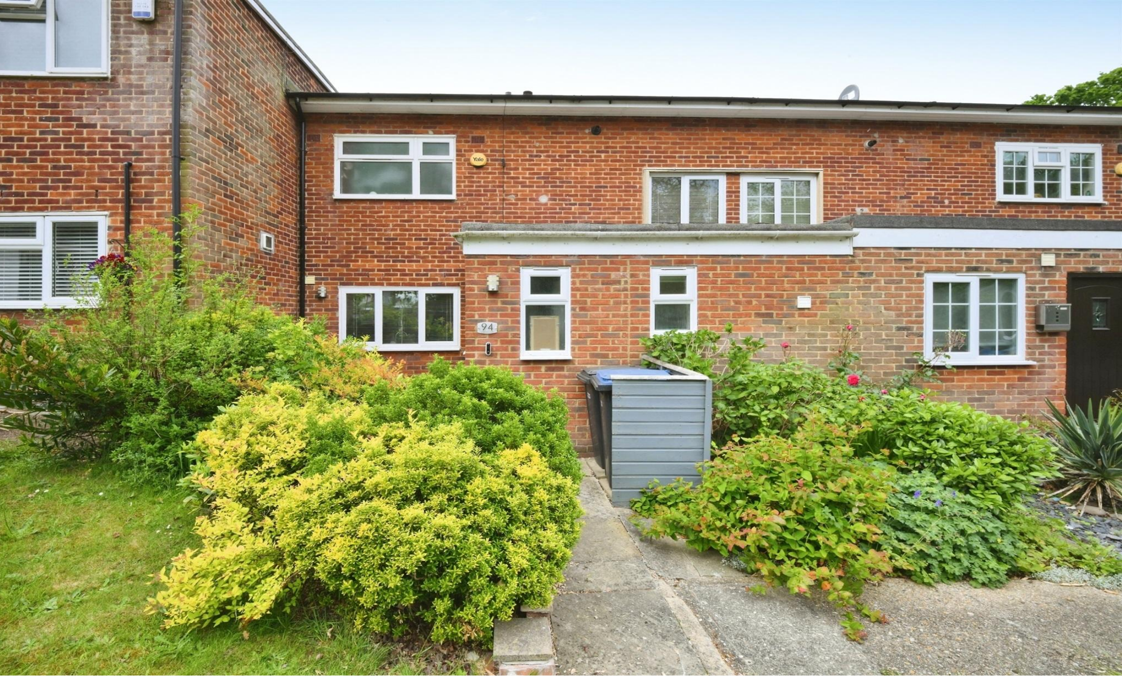
Glebelands, Harlow CM20 2PE
