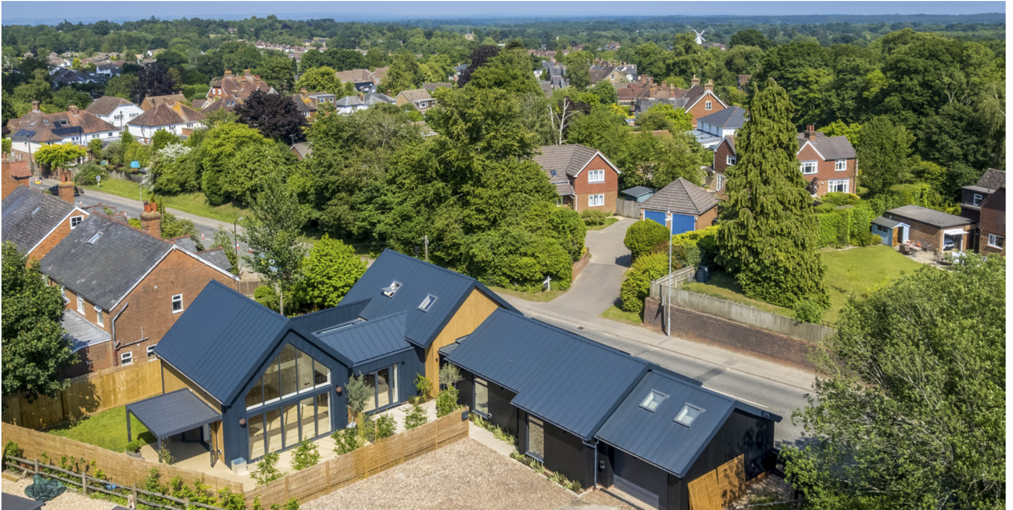
LARCH HOUSE Angley Road, Cranbrook, Kent
