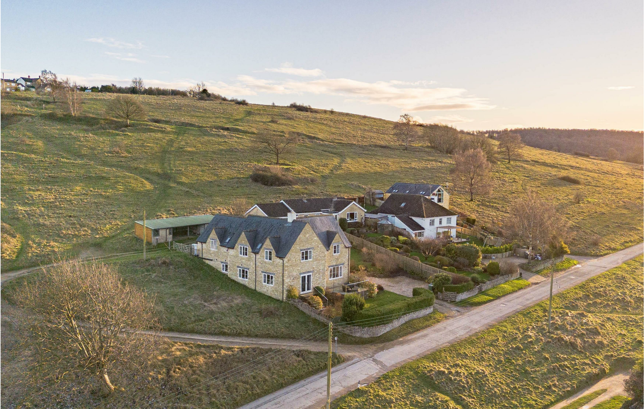
Aerial view of Hillside in Cranham
