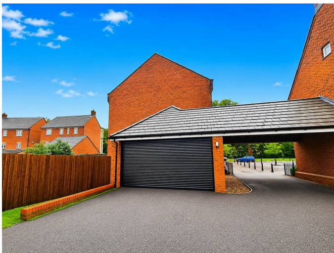
Garage and Driveway
