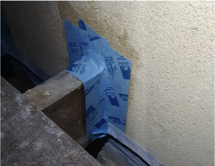
Airtight taping of joists using proprietary (age tested) airtightness products. Importantly, the lime plaster has been continued through the joist zone.
