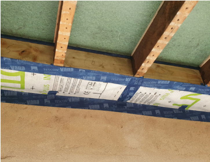
Airtight taping at roof eaves using proprietary (age tested) airtightness products.
