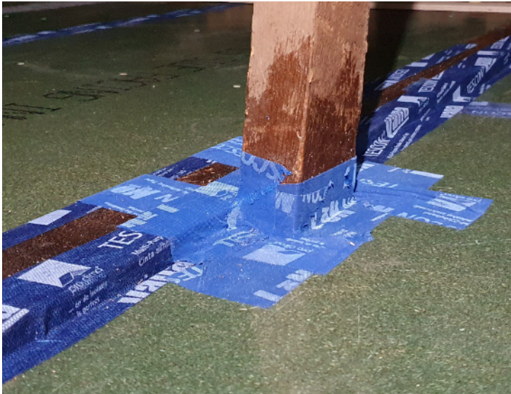
Airtight taping to loft deck using proprietary (age tested) airtightness products. As seen in this image, timber was primed to ensure good adherence.
