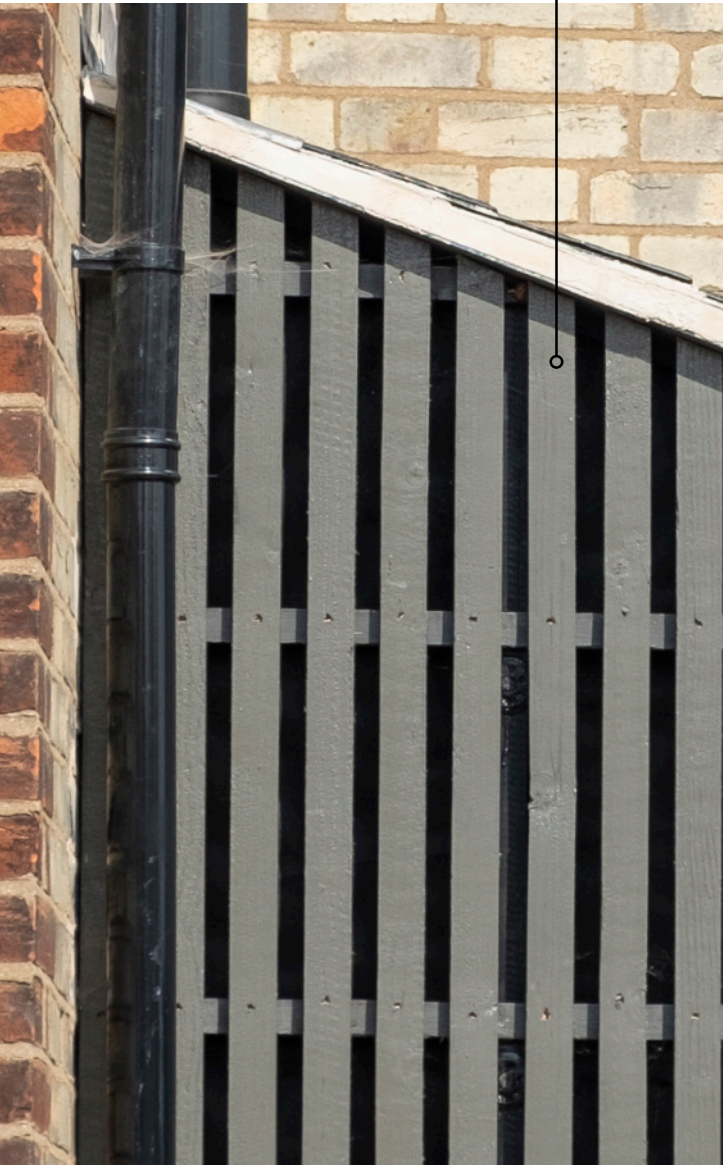
Roof Batten Cladding
