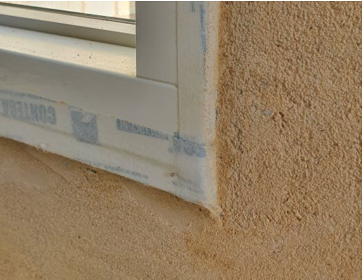
Airtight taping of windows using proprietary (age tested) airtightness products..
