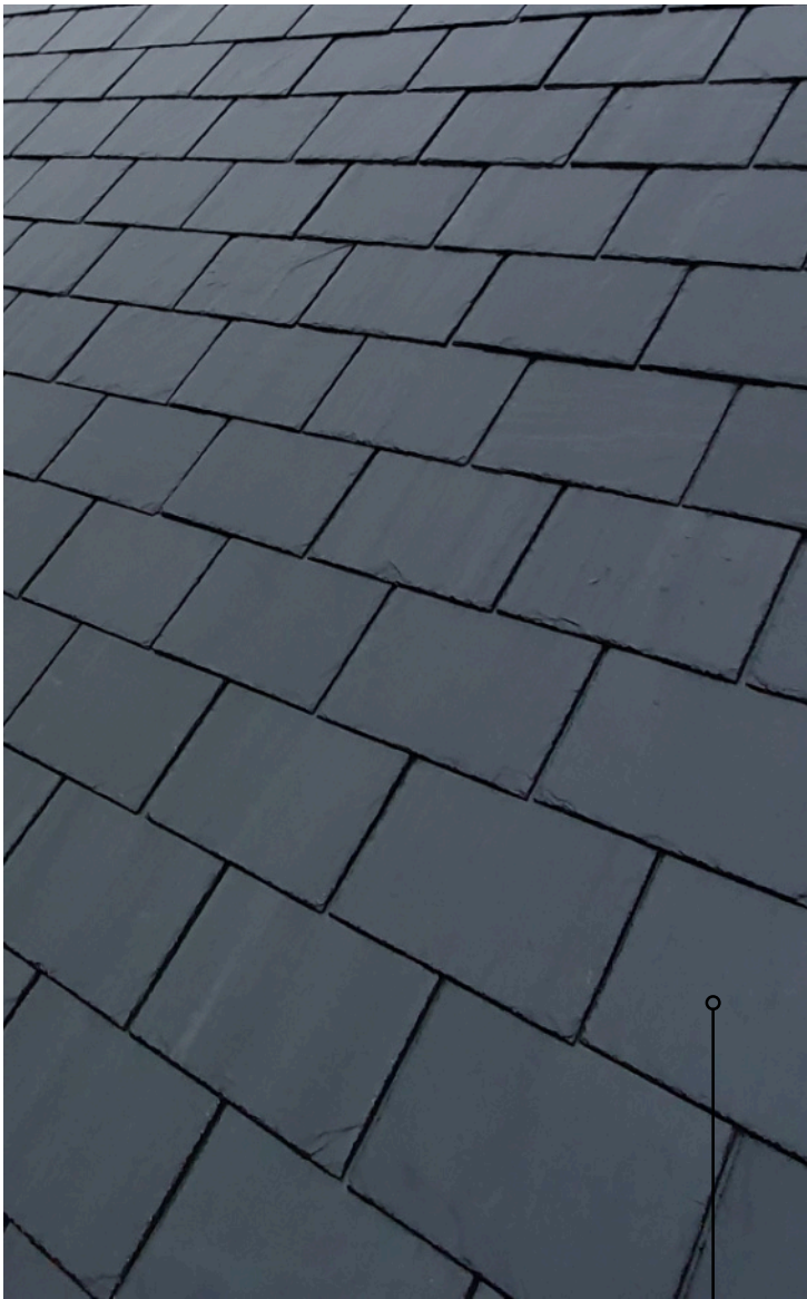
Completely Re-Roofed in Natural Slate
