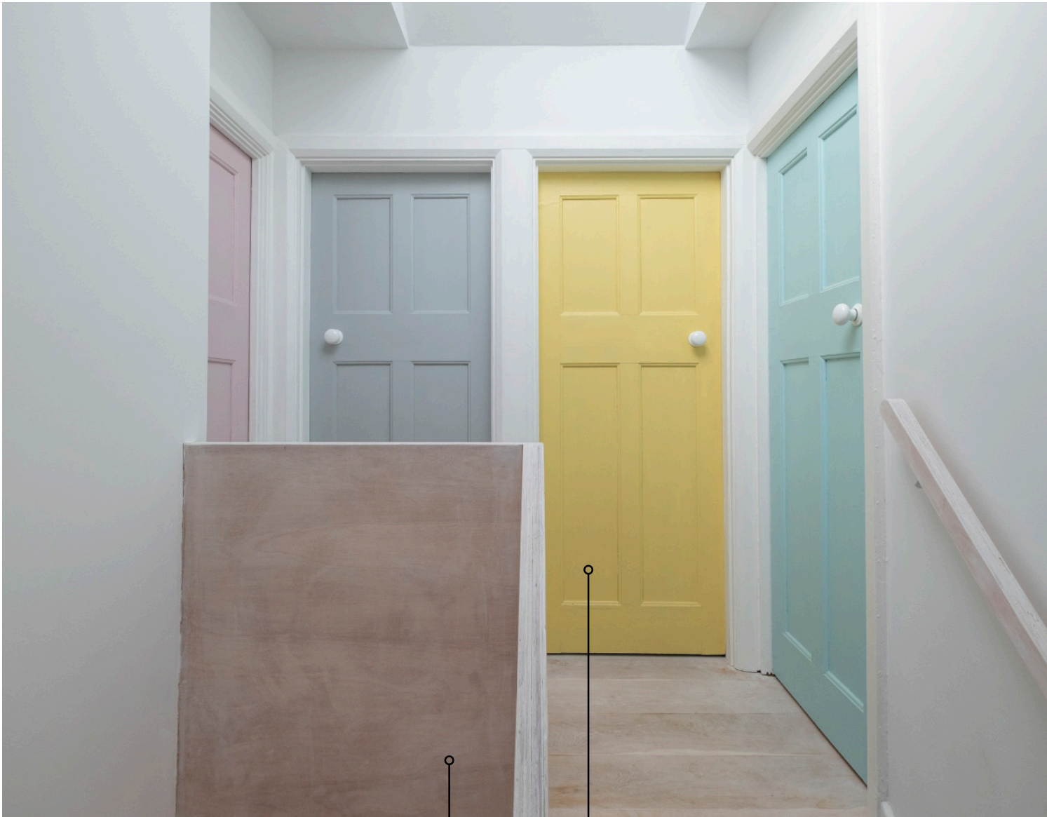
Plywood Stair Guarding & Handrail
