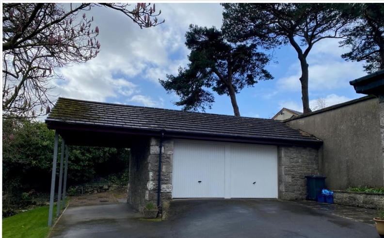
Garage to the right
