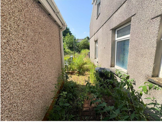
Garden overgrown and in need of attention.
