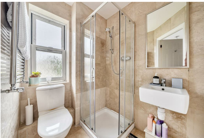
Double glazed window, W.C hand basin, shower cubicle, radiator.
