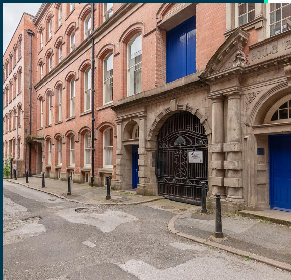
Mills Building, Plumptre Place, Nottingham, NG1
