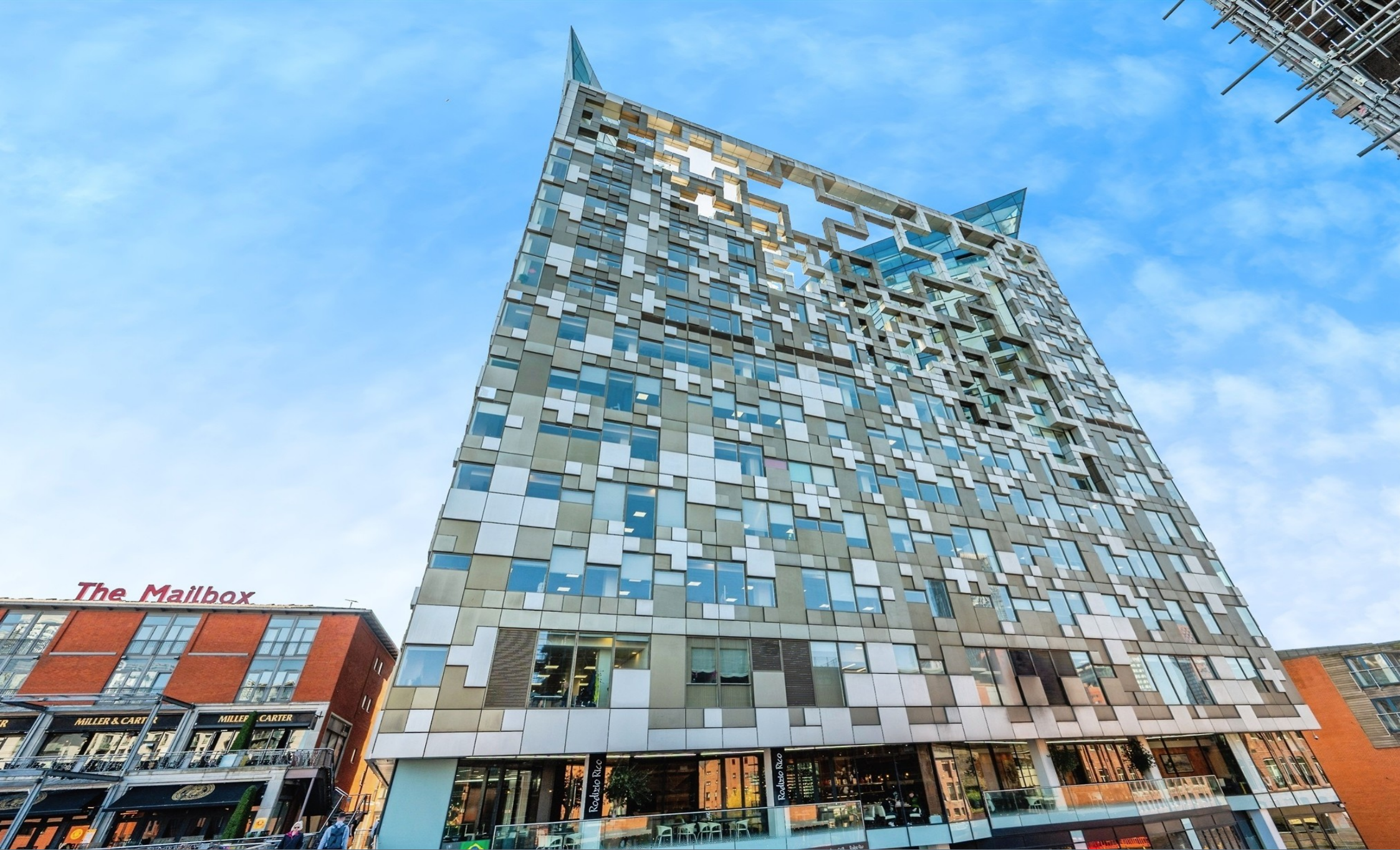
The Cube East Wharfside Street Birmingham
