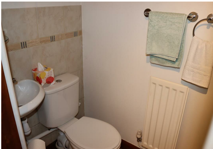
Ground Floor Shower Room
