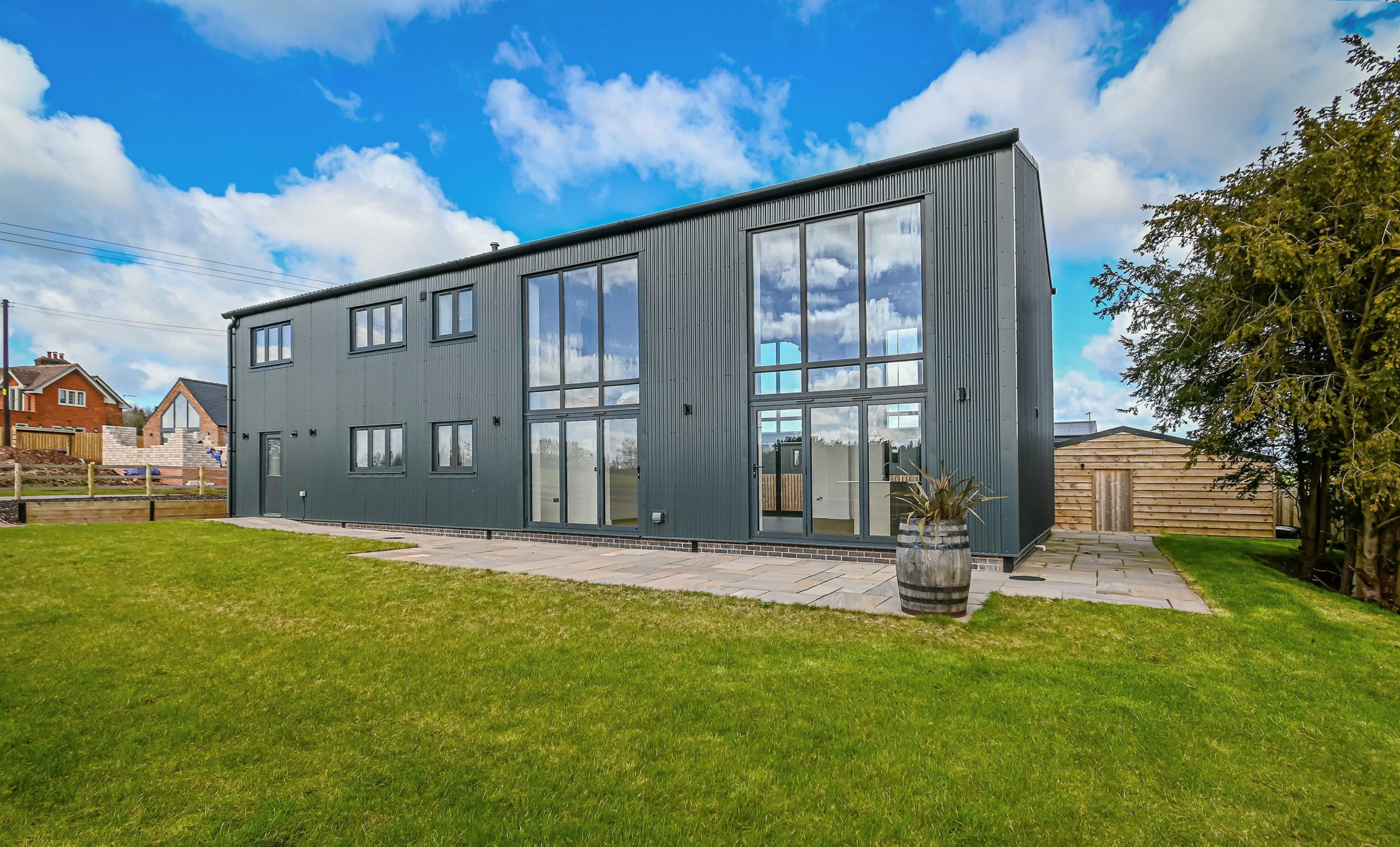
Coppice View Barn Glazeley, Glazeley, Bridgnorth, Shropshire, WV16 6AB
