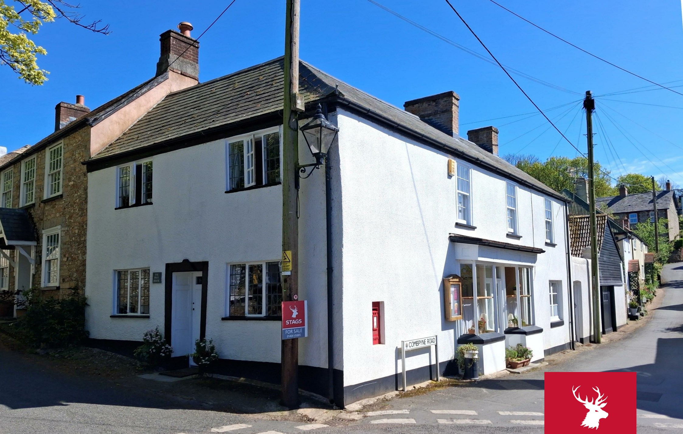
The Post House, Church Hill
