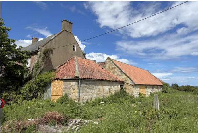
Building 2 (58' x 22' ext) forming the east side of the courtyard. This building has been re-roofed.
