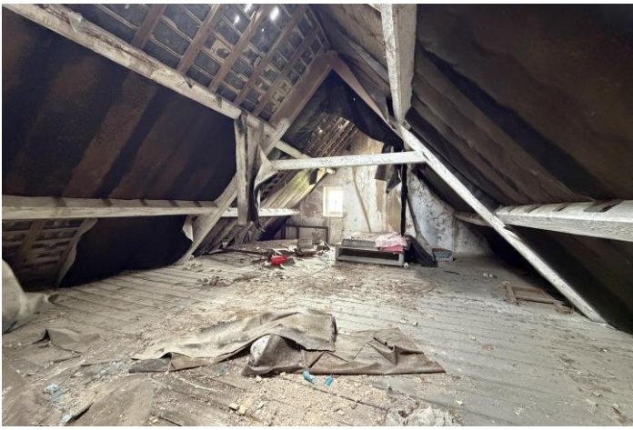
Attic Room 2 – A larger attic with exposed beams. This room, previously a bedroom, has a window in the east facing gable.
