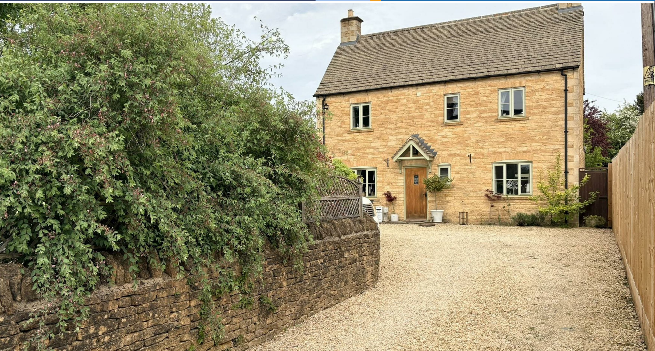
Jacobs House, Station Road , Bourton-On-The-Water, GL54 2ER Guide Price £710,000
