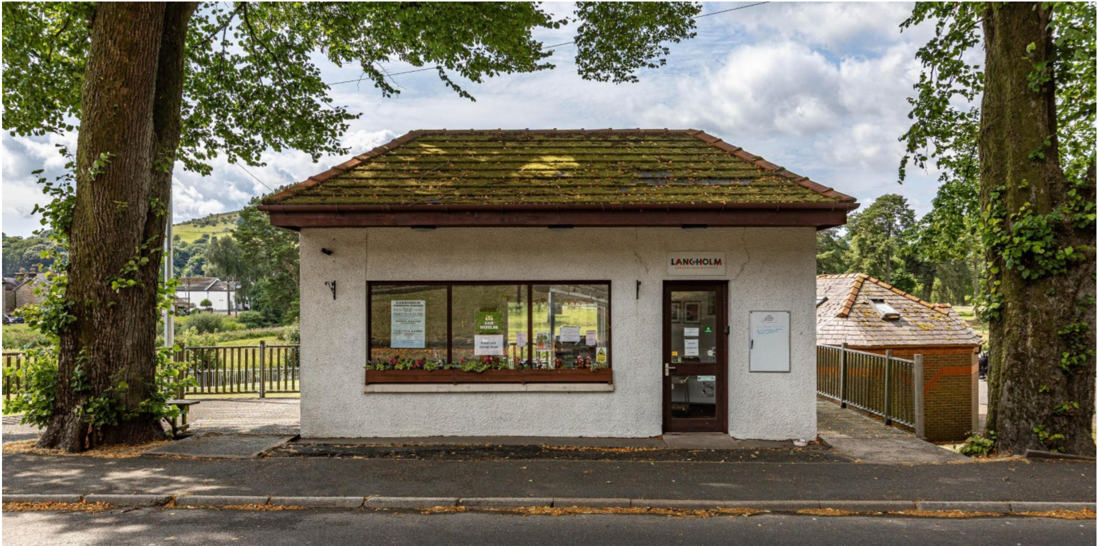
Commercial Premises - The Kiosk, Townhead, Langholm, DG13 0EP
