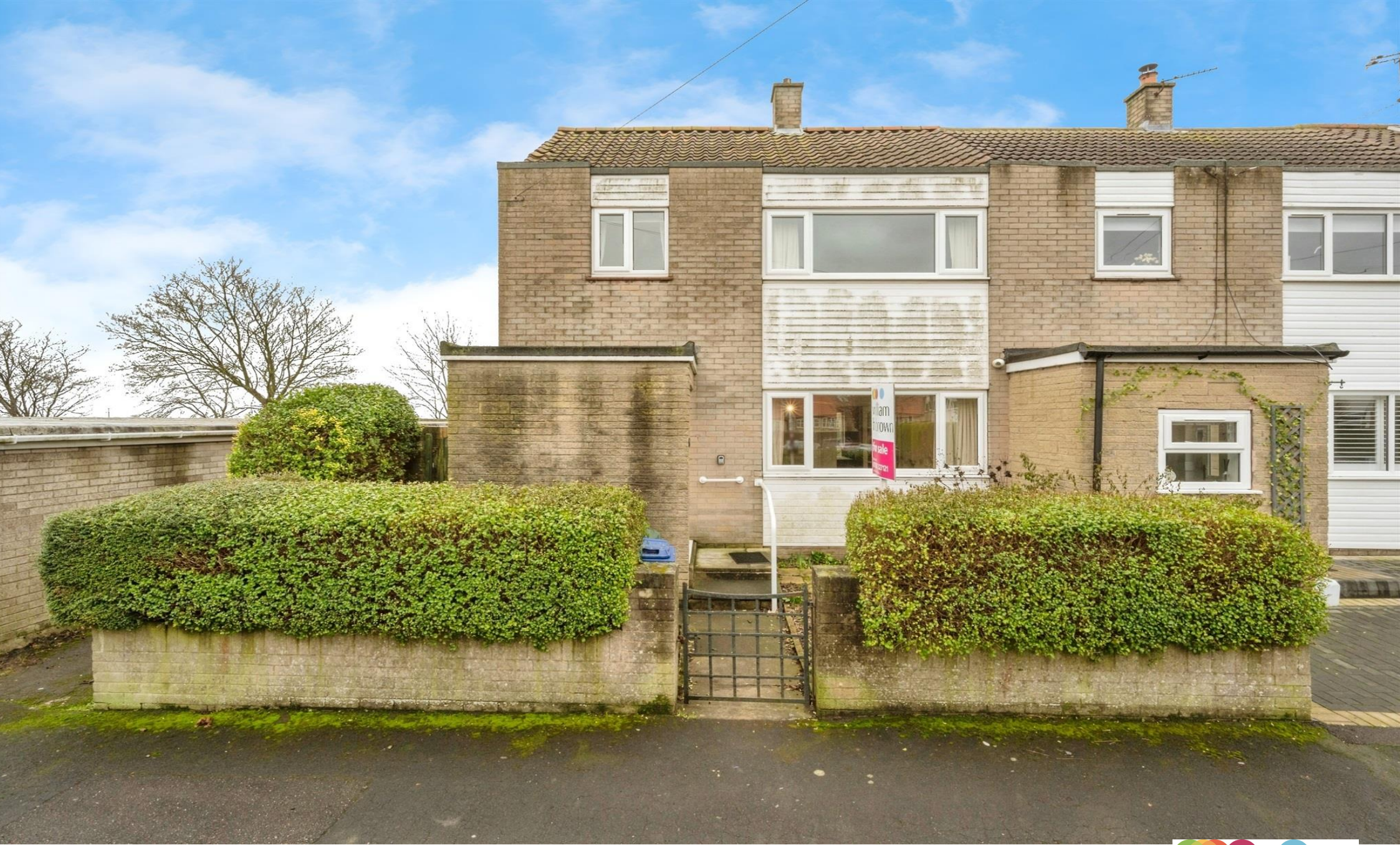
Church View, Wadworth Doncaster
