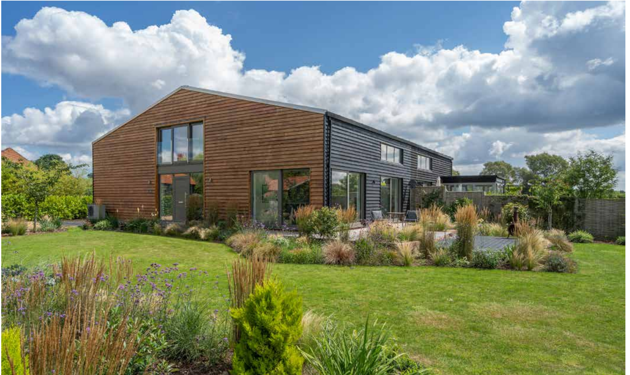
Westside Barn Yarmouth Road | Kirby Cane | Norfolk | NR35 2HJ
