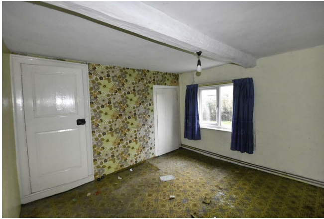
Boxed in fireplace, radiator.
