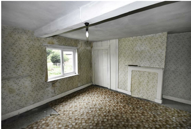
Built-in cupboard, radiator.
