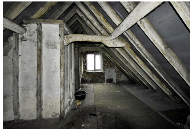
Attic space with gable window, attic store.
