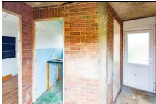
Outbuilding Covered Alley
