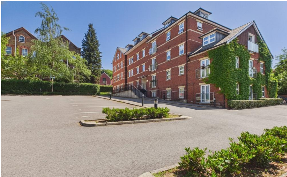
Carpenters Court, 151 Croydon Road, Caterham CR3 6PX
